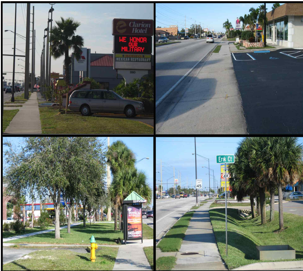
Figure 2. Typical conditions of sidewalks
